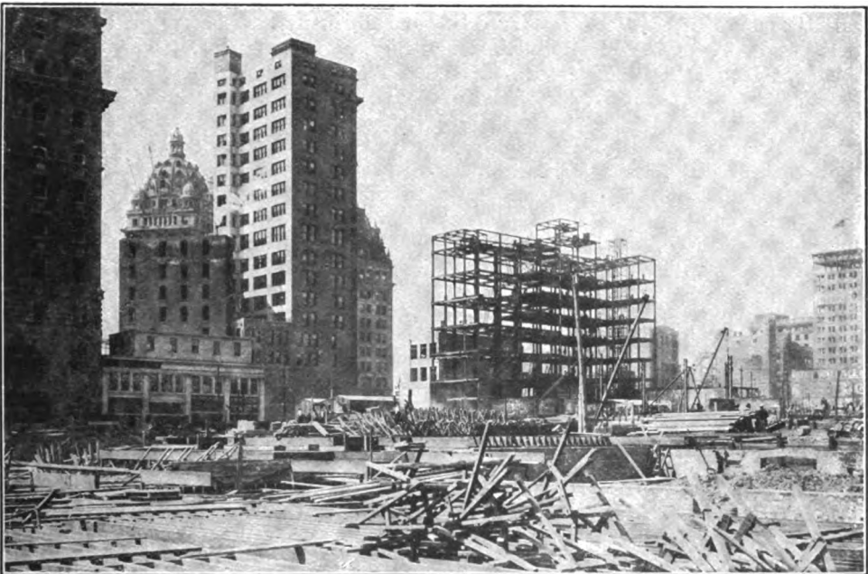
RECONSTRUCTION WORK IN THE HEART OF THE CITY
